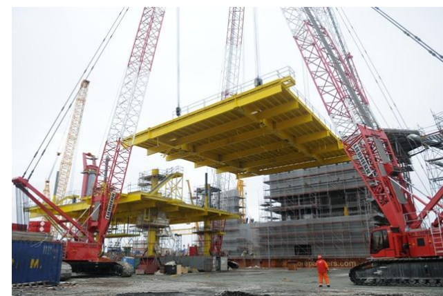
Works performed on Akcakoca Project
